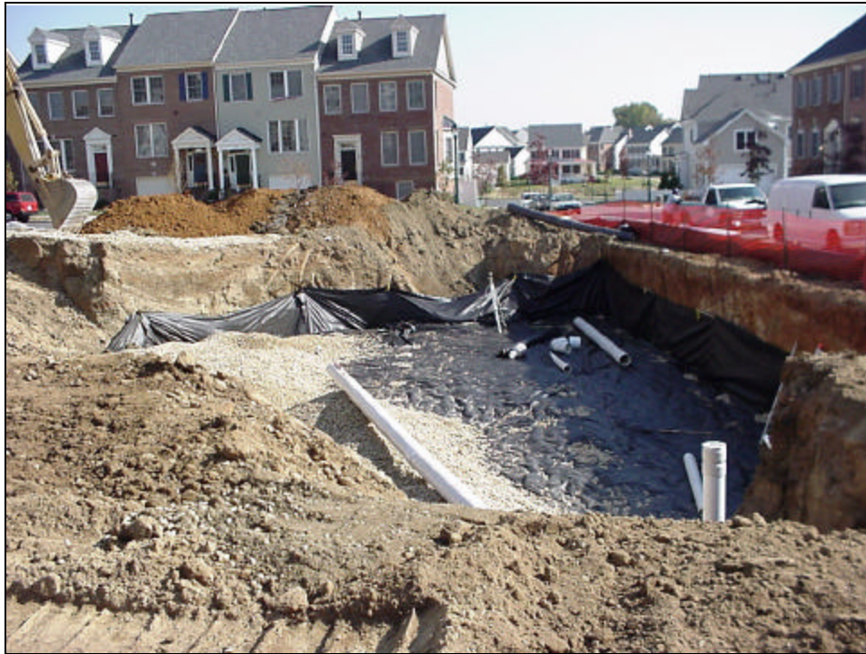
Figure 15. Sand Filters construction in Pocket Park
